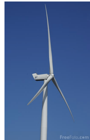
Horizontal Axis Turbine
